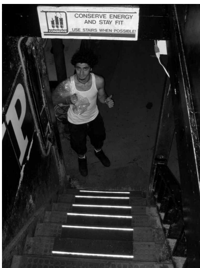
Summer Social Chair A.J. "Bootz" Chammas admires the new treads the basement stairs
